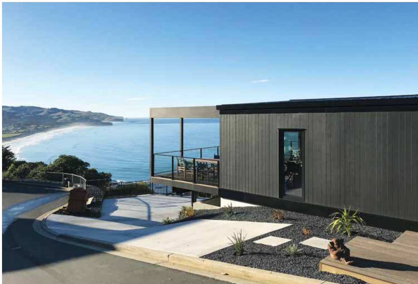
WD Homes specialises in challenging builds whether on steep sections or complex architectural designs.
